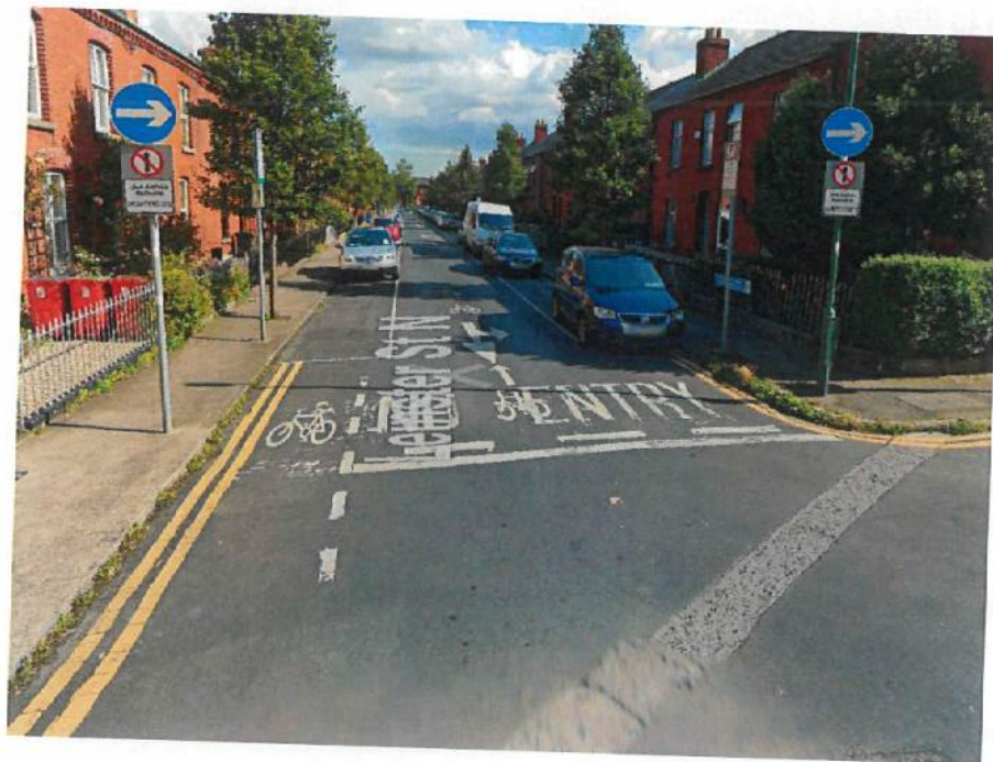
Contraflow cycling in Dublin: Description Junction of Leinster St and Ulster St looking east - There is a no-straight ahead sign with an exemption plate for cyclists. The no-entry markings are interrupted by a short length of on-road cycle track. Picture from Google Streetview
