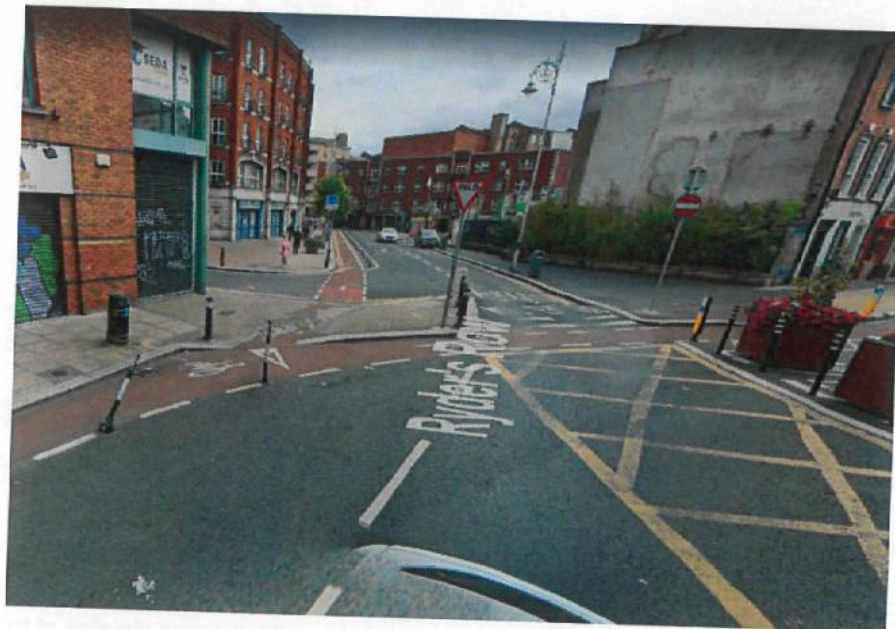
Contraflow cycling in Dublin: Description Junction of Capel St and Ryders Row looking south east. Ryders row is two-lane with a contraflow cycle-track. Picture from Google Streetview.
