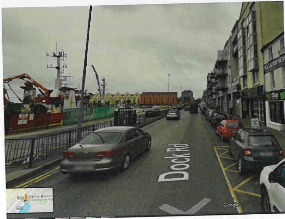
Google Streetview Image of Dock Road in Galway: Note the hostile railings at the road edge. This is part of a cycling hostile one-way system. Under the Galway Transport Strategy and Bus Connects proposals, this is one of only two routes by which people on bicycles might access the old core of the city from the east. This is also the only direct route to locations like the Claddagh and the West End/Dominick St area.
